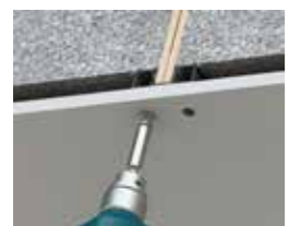
Dry wall bit assembly
