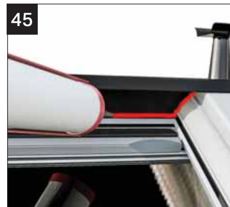
45 Seal around the top of each glazing bar top capping where it meets the rain baffle. Next, run a bead of sealant along the edge where the glazing meets the rain baffle.
