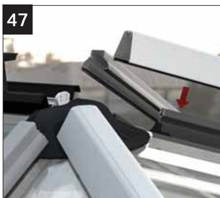
47 Install bar caps, securing flashing into place. Point around bar caps.
