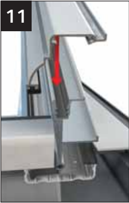
Fit the starter bar top capping in position.
