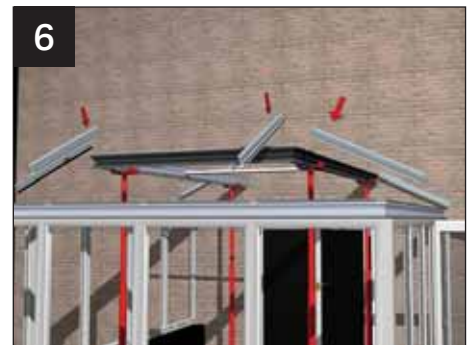
6 Now the Lantern eaves beam is assembled into a one piece structure, temporarily support it. Attach the glazing bars according to the component location plan. Tighten the bars, at the pagoda beam end first and then at the main eaves beam second.
