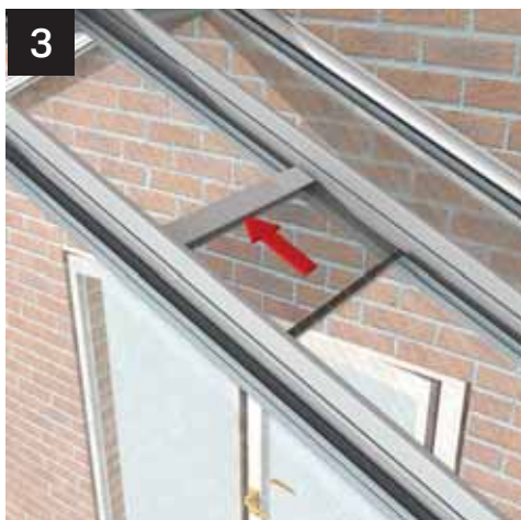
Fit lower glass unit into glass jointer.
