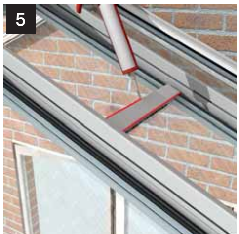
Using appropriate sealant run beads along the top and bottom of the glass jointer.
