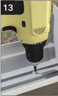
Secure in place using screws provided with cap covers.
