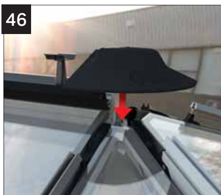
Apply silicone to weather seal as shown. Apply weather seal to glazing, locking wings around ridge - remember, MS Polymer for self cleaning glass (see p38).
