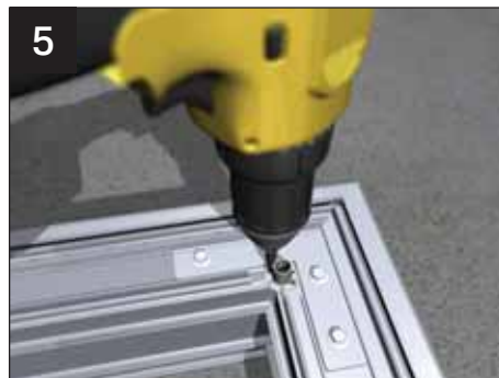
5 If supplied, fasten to each corner the tie bar drop rod fixing bracket to the underside of the lantern eaves beam.
