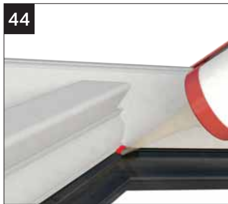
44 Carefully point the corners on each side of the capping where the gaskets abut each other
