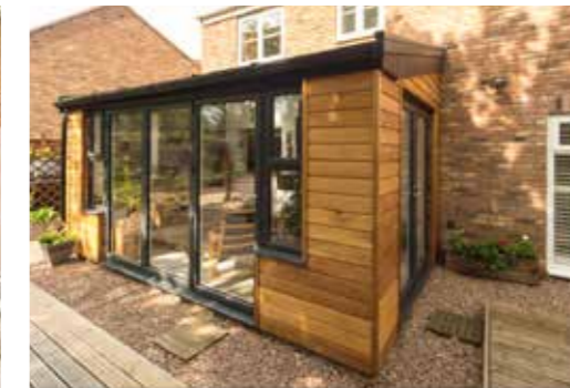
Horizontal Timber Boards
