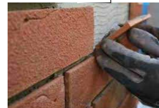
Brick Slips Application
