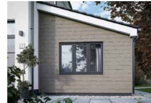
Horizontal Cement Boards
