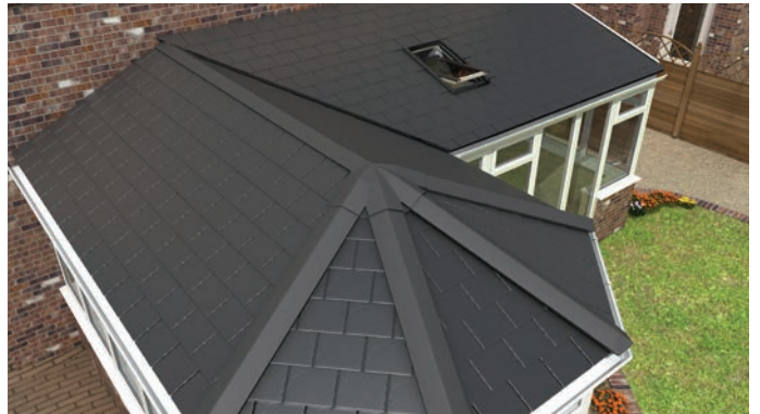
Chosen tile is added ensuring weathertightness and the gutter and external trim are secured in place.
