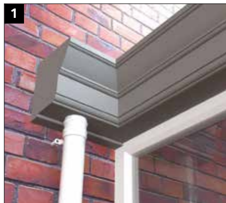
1 Return Cornice and guttering along house wall.
