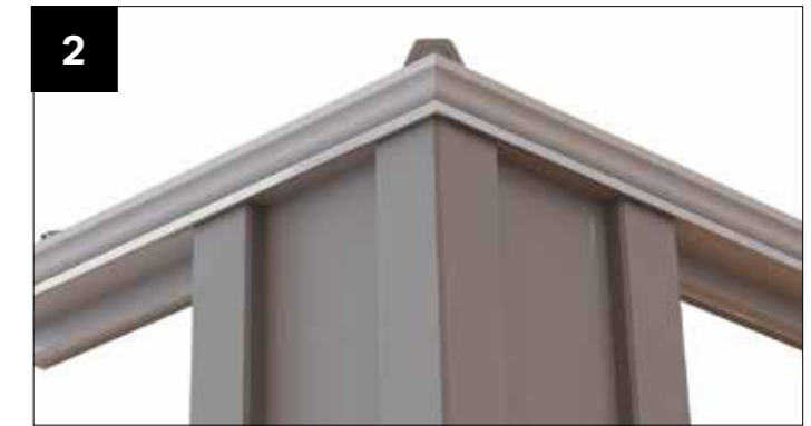
2 Super-insulated columns with Cill
